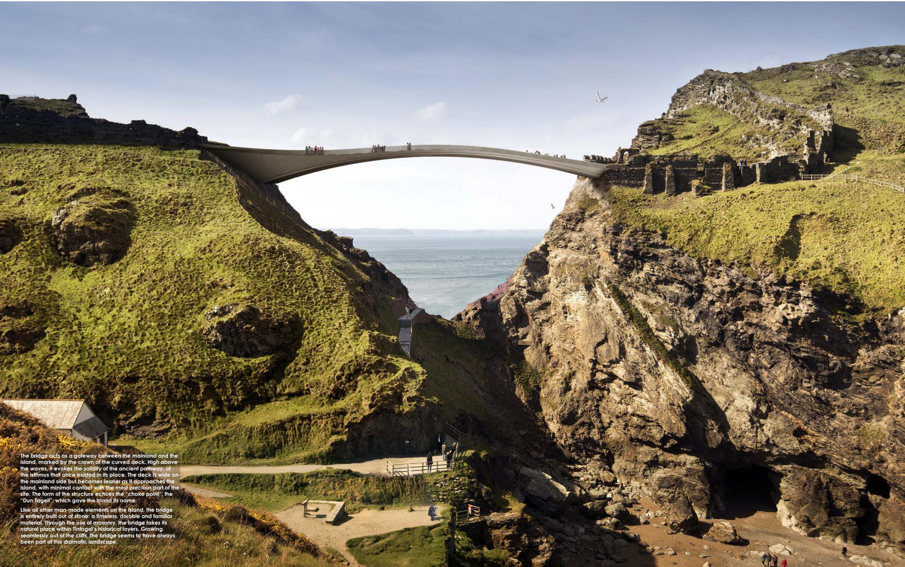
The bridge acts as a gateway between the mainland and the island, marked by the crown of the curved deck. High above the waves, it evokes the solidity of the ancient pathway, of the isthmus that once existed in its place. The deck is wide on the mainland side but becomes leaner as it approaches the island, with minimal contact with the most precious part of the site. The form of the structure echoes the "choke point", the "Dun Tagell", which gave the island its name.
