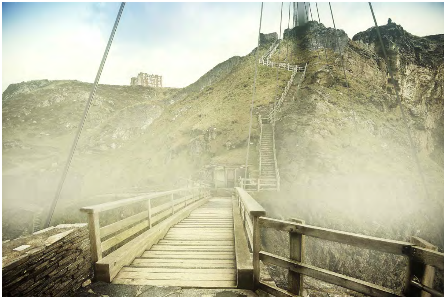
VIEW FROM THE LOWER LEVEL TOWARDS THE LANDING OF THE NEW LIGHTWEIGHT AND TRANSPARENT BRIDGE
