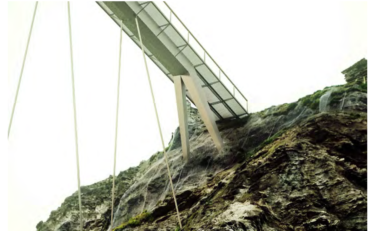
INCLINED PILLARS ON THE ISLAND SIDE, REDUCING ARCHAEOLOGICAL IMPACT
