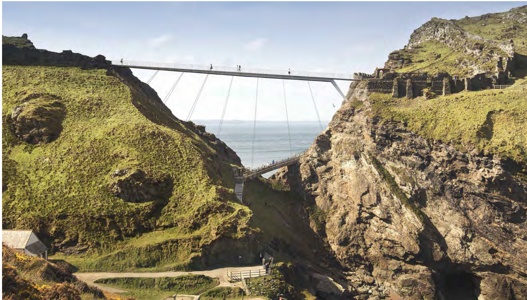
A BRIDGE PRESTRESSED BY STAINLESS STEEL PLATES ANCHORED IN THE RAVINE, EAST ELEVATION
