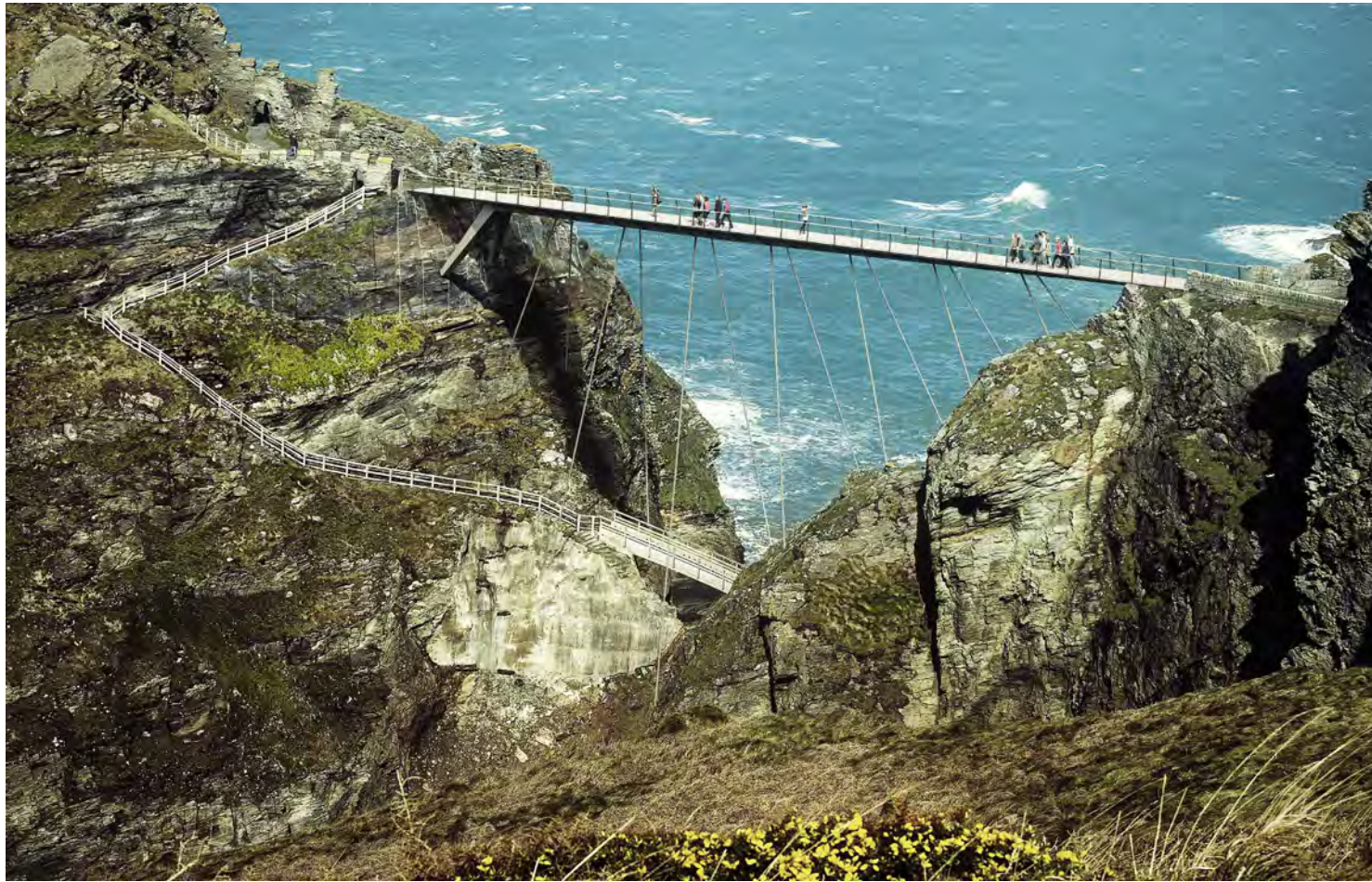
REESTABLISHING THE HISTORIC WALKWAY TO THE ISLAND, FILLING THE VOID WITH PRESTRESSED STEEL PLATES. VIEW FROM THE SOUTH-WEST COASTAL PATH
