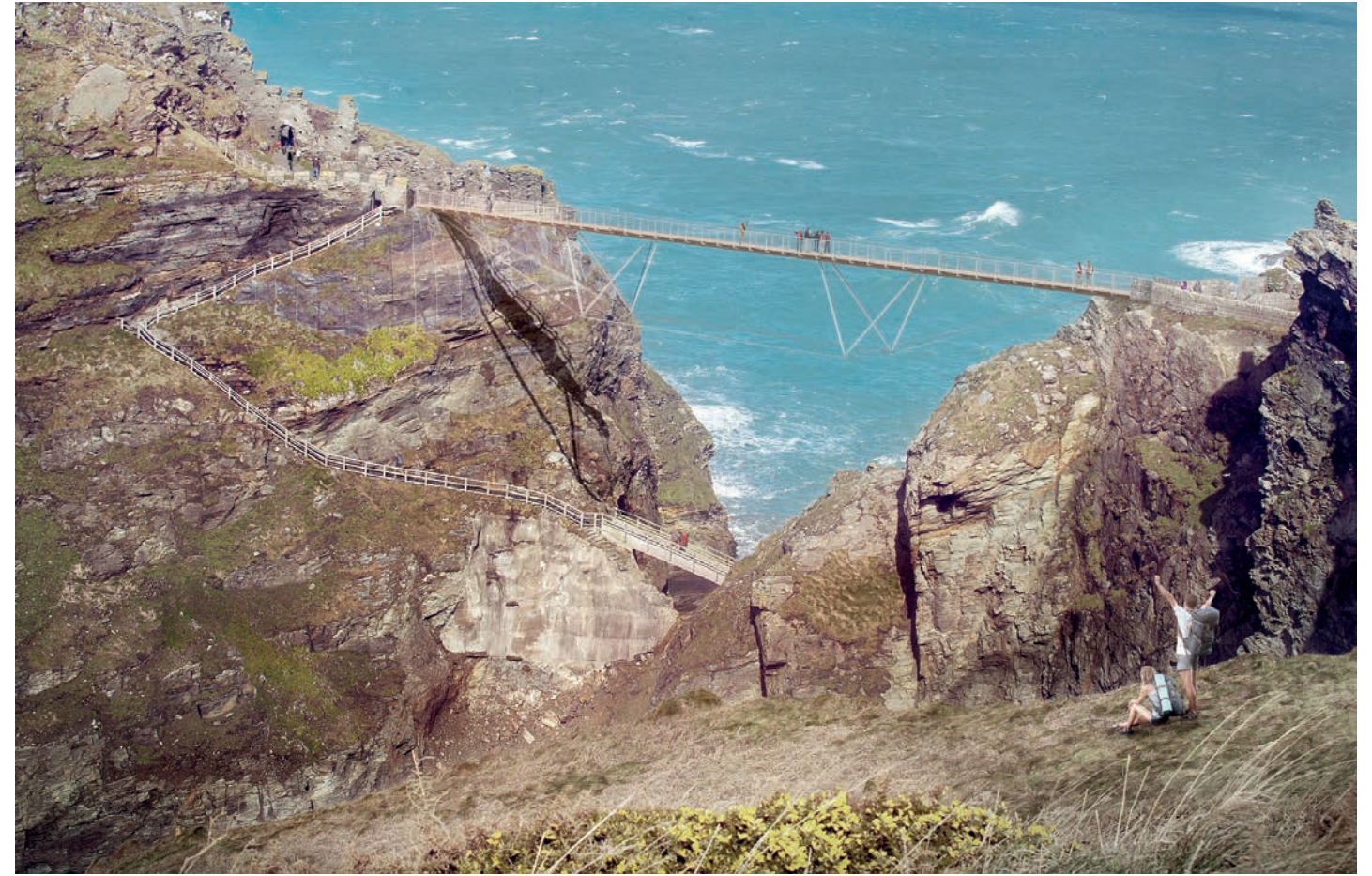
View of bridge looking north
