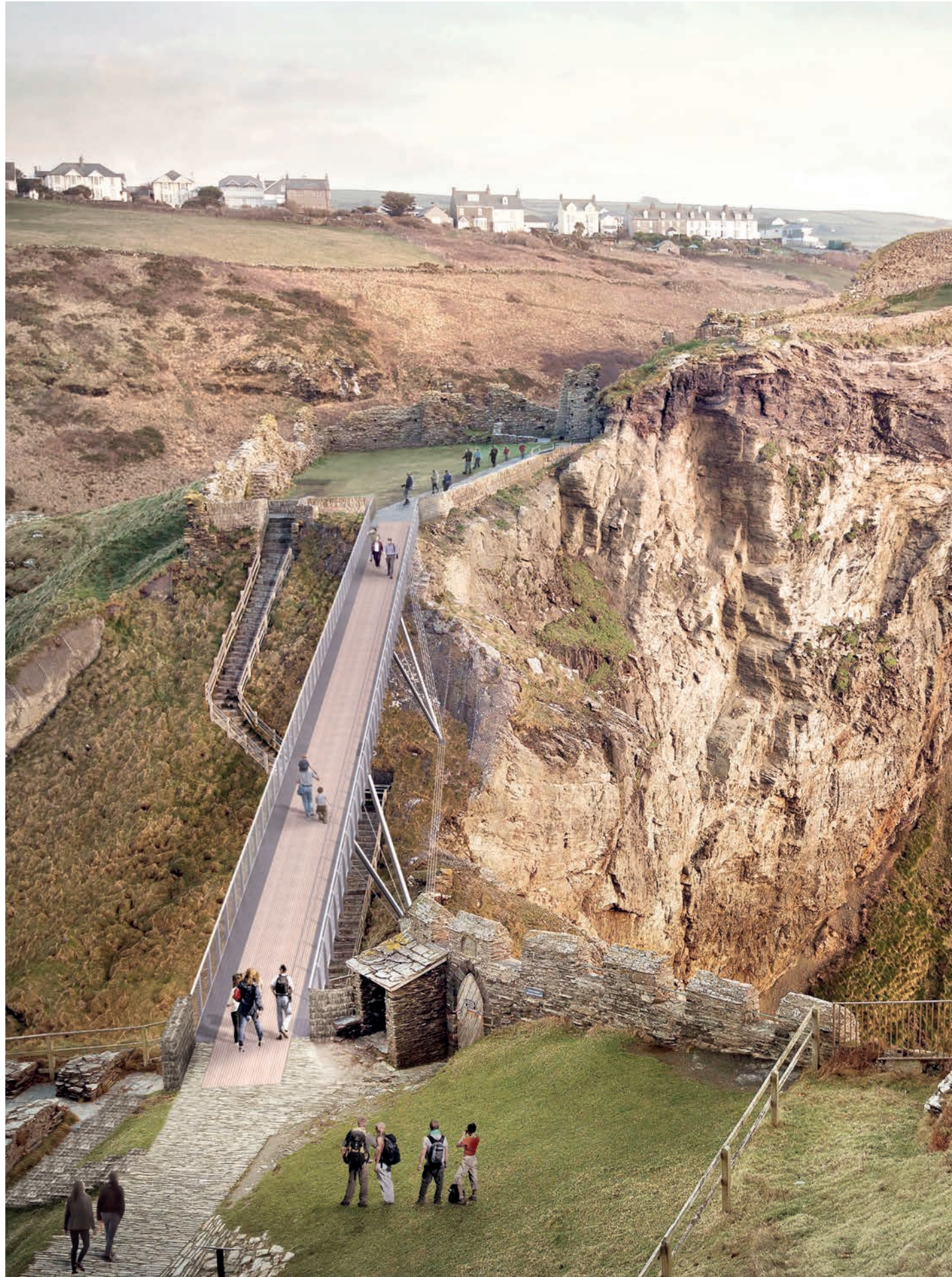
Elevated view of bridge looking southeast
