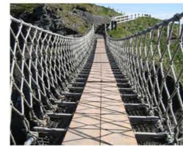
Carrick-a-Rede Rope Bridge, N.Ireland
