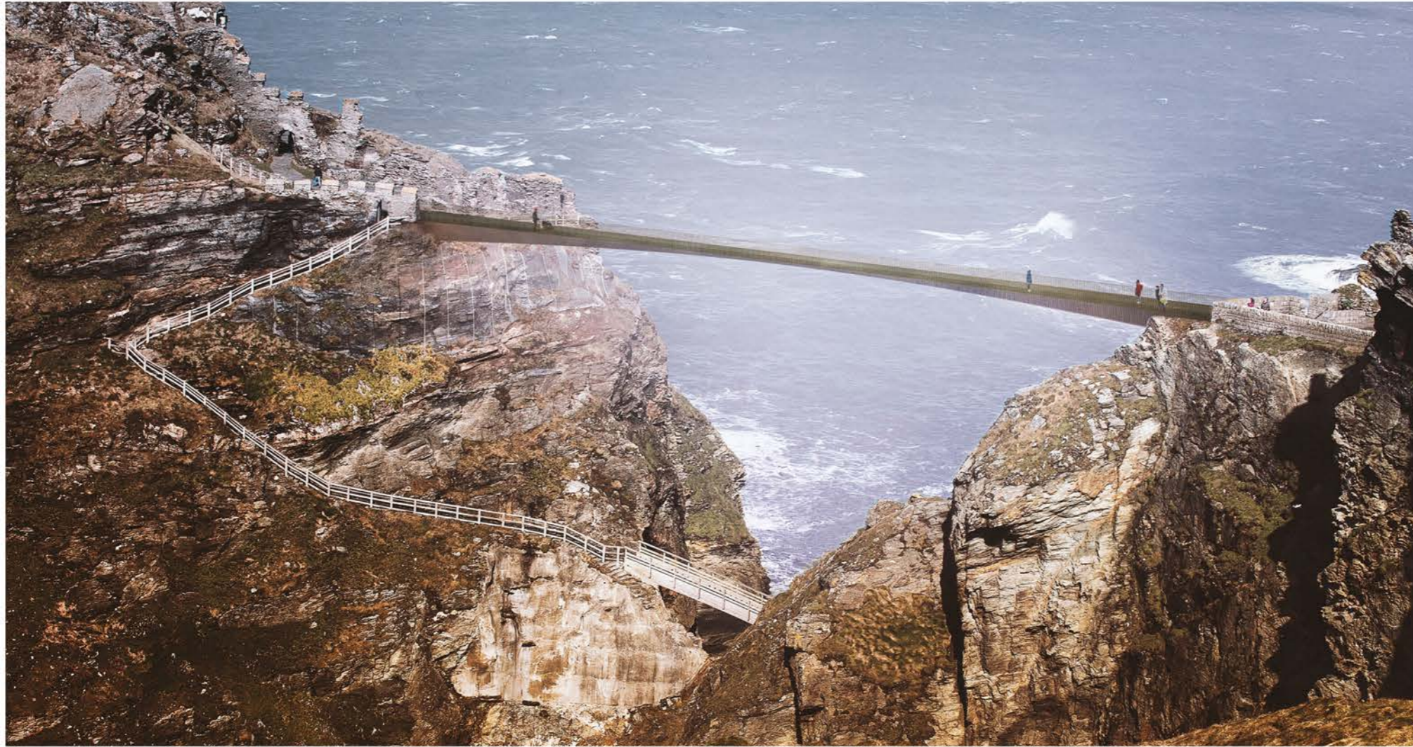
West Elevation from Mainland
